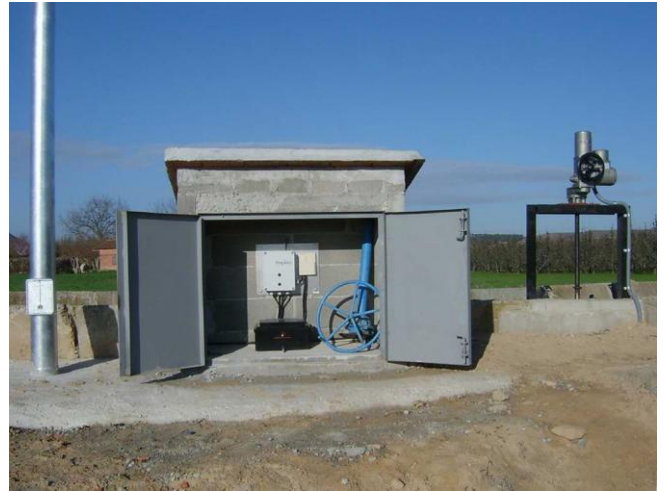
A retrofitted solar powered low voltage installation, with a Centork DC actuator fitted to an existing penstock, replacing the original handwheel awaiting disposal in the new control cabinet.
