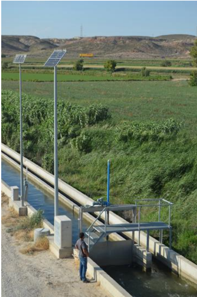
Typical solar powered remote penstock installations equipped with 24VDC Centork actuators (Courtesy of Riegosalz)
